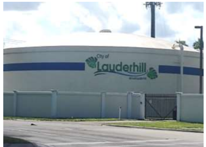
Security upgrades such as concrete walls and fences will continue to protect and ensure the City's water supply
