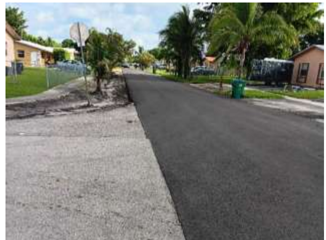
Roadways are resurfaced on a schedule for safety and to reduce repair costs. Area at NW 17 Court shown above.
