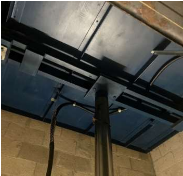
Replacement of the Sadkin Center elevator
