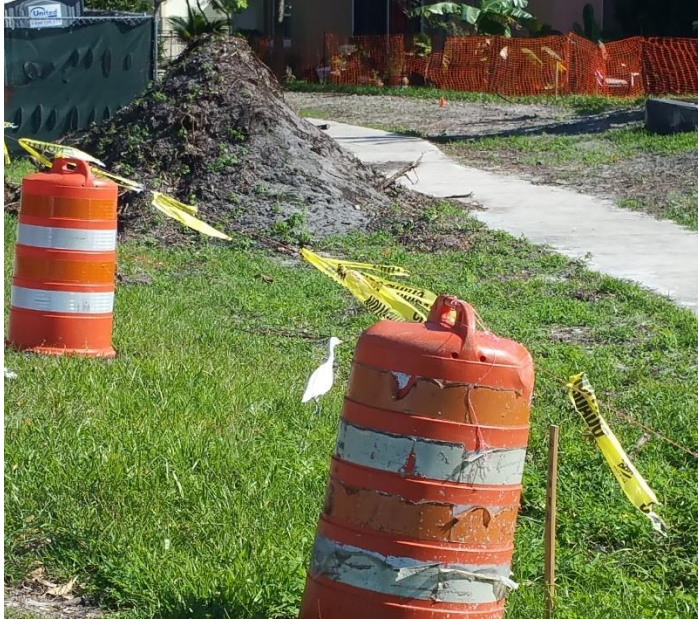
West Construction has begun work on installing walls
