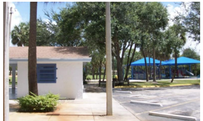
The Community Center will be renovated along with numerous improvements to the park amenities
