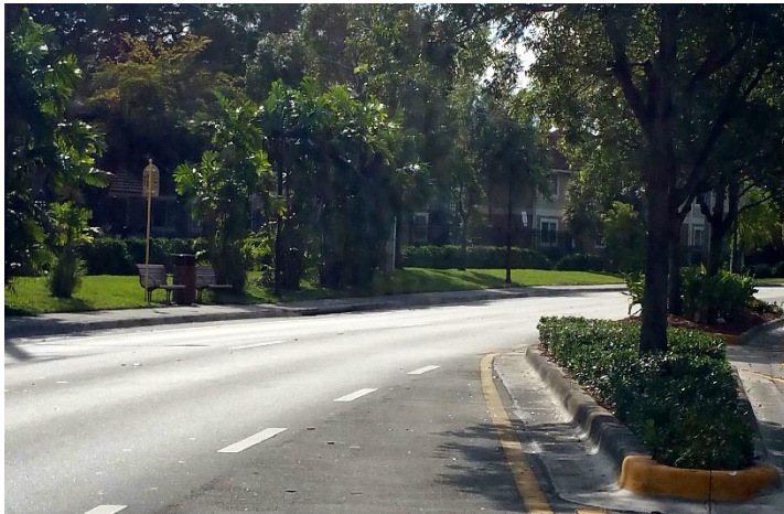
The NW 56 Avenue project from the 2005 GO Bond will be a model for the work planned for NW 47 Avenue
