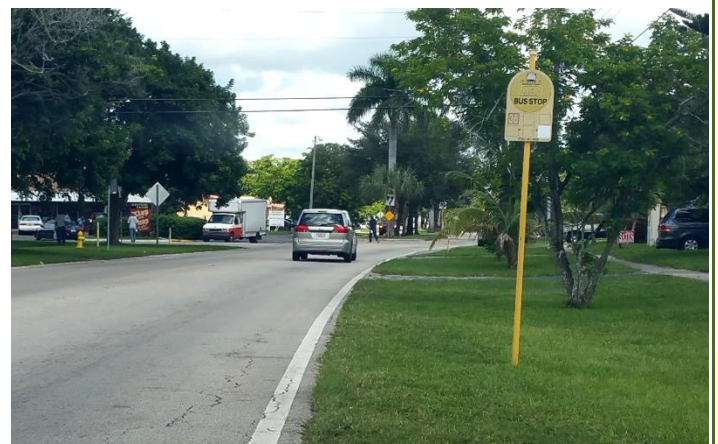
The renovation design for NW 47 Ave is challenging because of the limited right-of-way available
