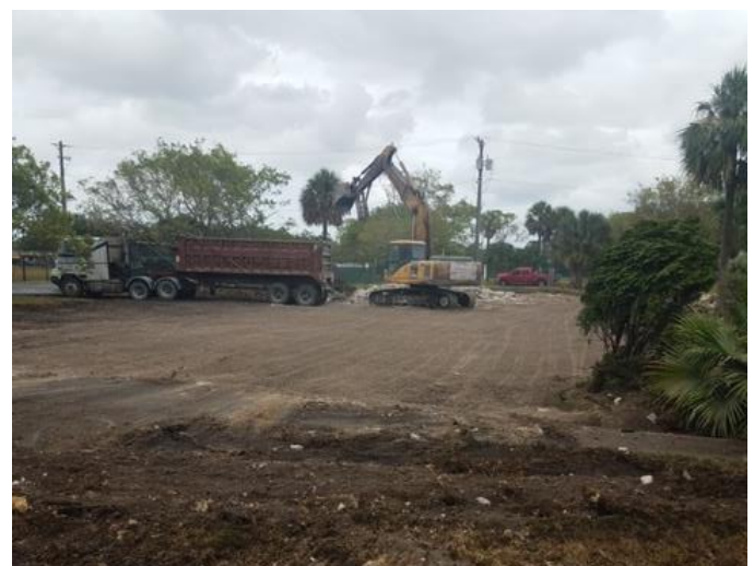
Demolition of St George church to allow for park expansion
