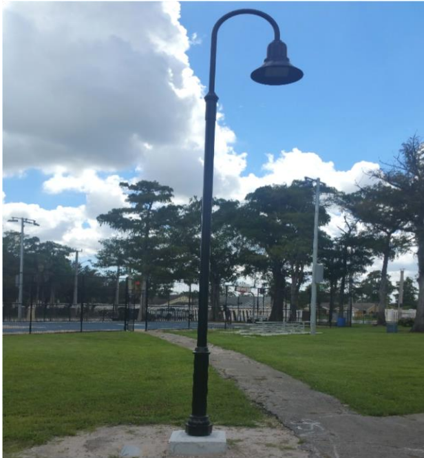
New pedestrian lighting installed at Gleason Park
