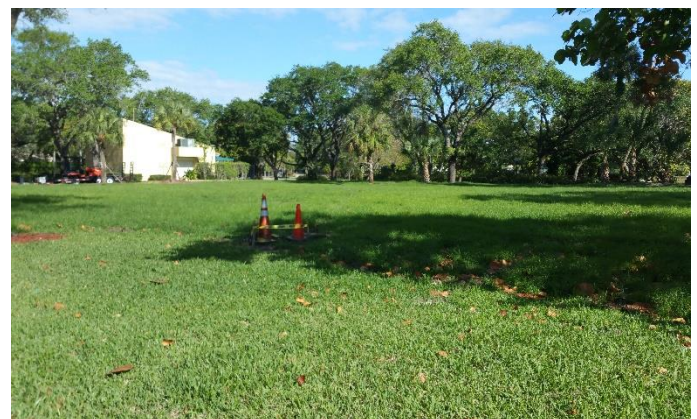
Demolition of the old Annex on NW corner of City Hall site was completed and site restored with sod and irrigation
