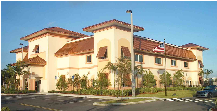
New Lauderhill Police Headquarters on Oakland Park Blvd.
